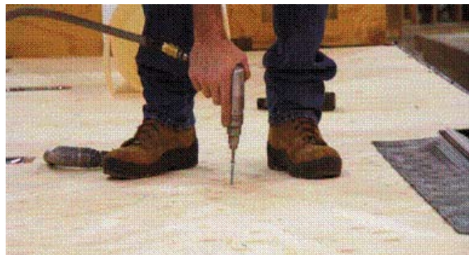
5/8" TONGUE AND GROOVE, MARINE GRADE PLYWOOD FLOOR
