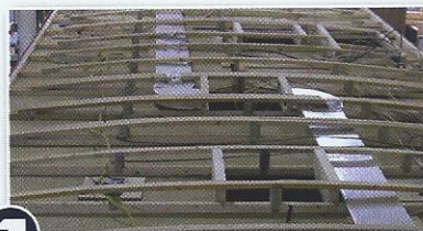
5" Roof Truss with Ducted AC and Walkable Decking
