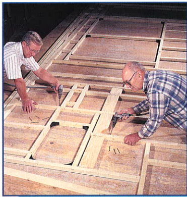
Glued and Screwed Construction on Complete Wood Super-structure (3 Year Warranty)
