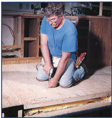
5/8" Plywood Flooring on 2x2 and 2x4 Framing (No Plywood Substitutes)
